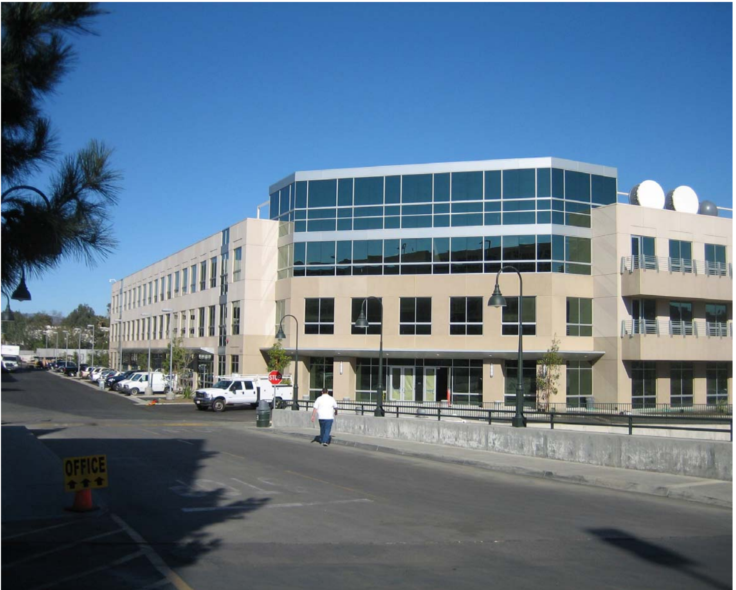
Main Entry Facade
